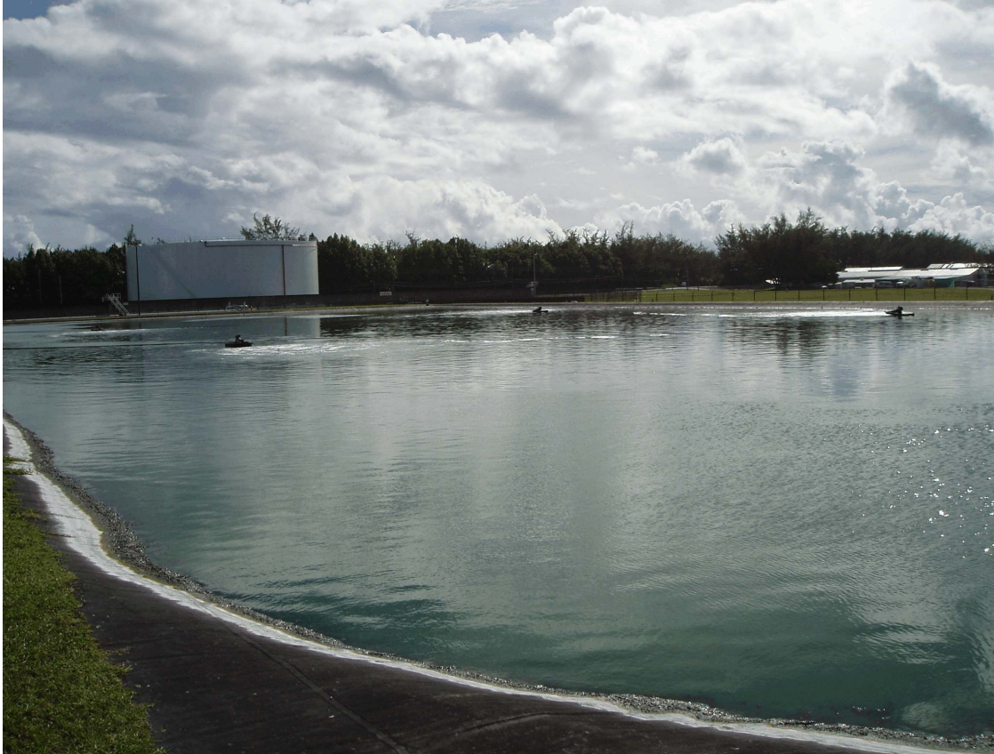
Secondary treatment aeration pool Diego Garcia
